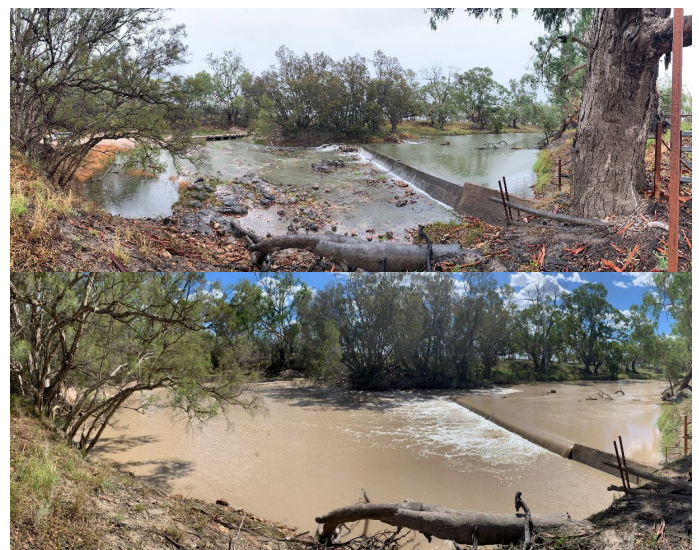
Before (top) and during (below) the flow at Mogil Mogil Weir. Photos: CEWO.
